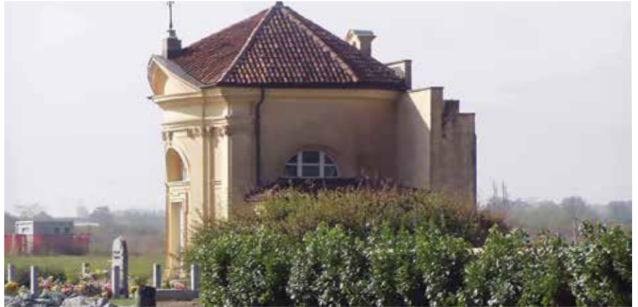
figs. 1-4. Cimitero Parco (Turin), view from inside (photos by AFC Torino s.p.a).
