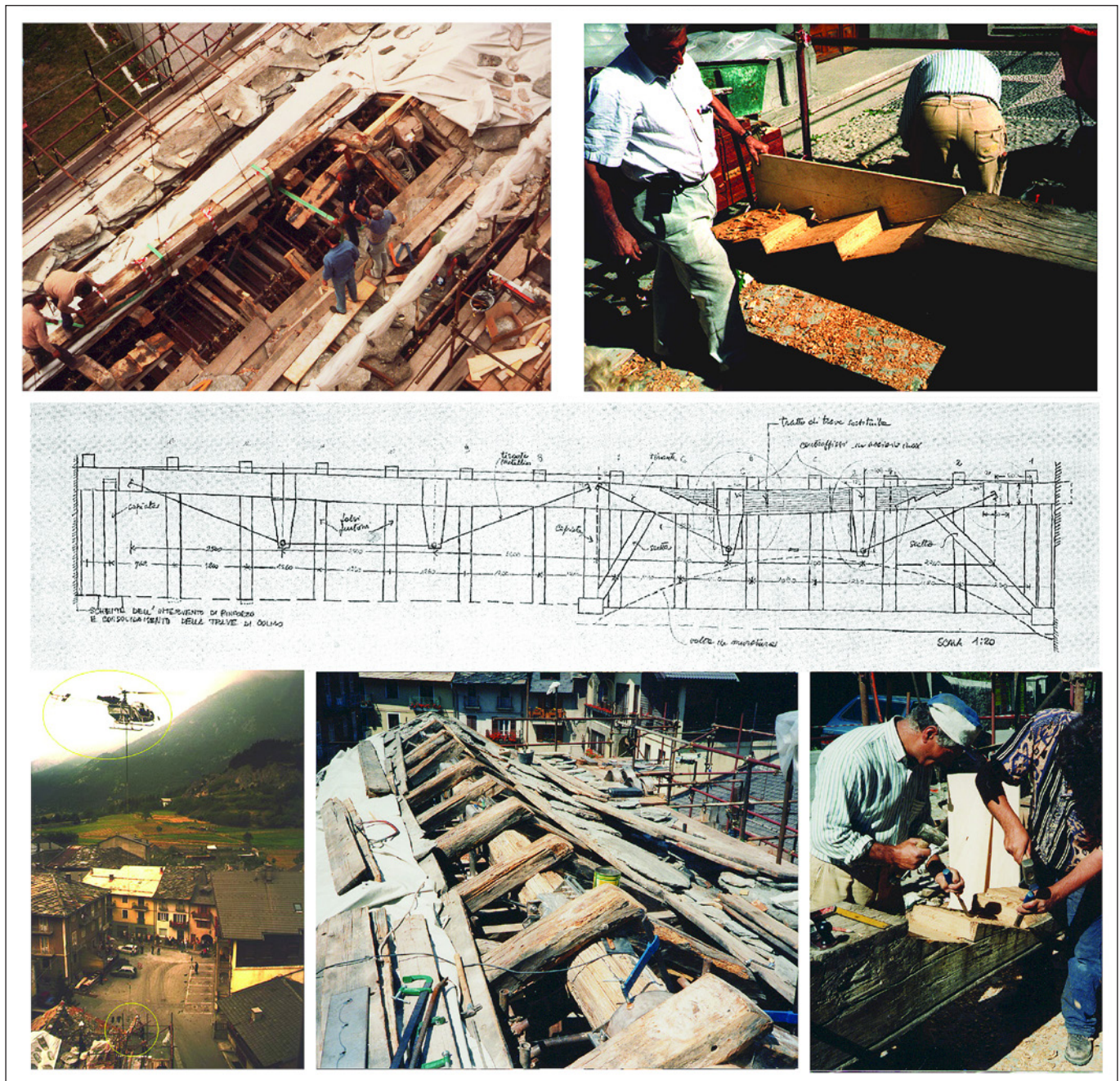
Fig. 10. Phases of the interventions carried out in 2000 with the integration of timber elements, the realization of the double “dart of Jupiter” joint, the transportation of the larch beam on the construction site, some details of the steel elements of the reinforced beam, and the scheme of the reinforcement intervention with Polonceau system. (Image source: drawings and photos courtesy of C. Bertolini-Cestari).
