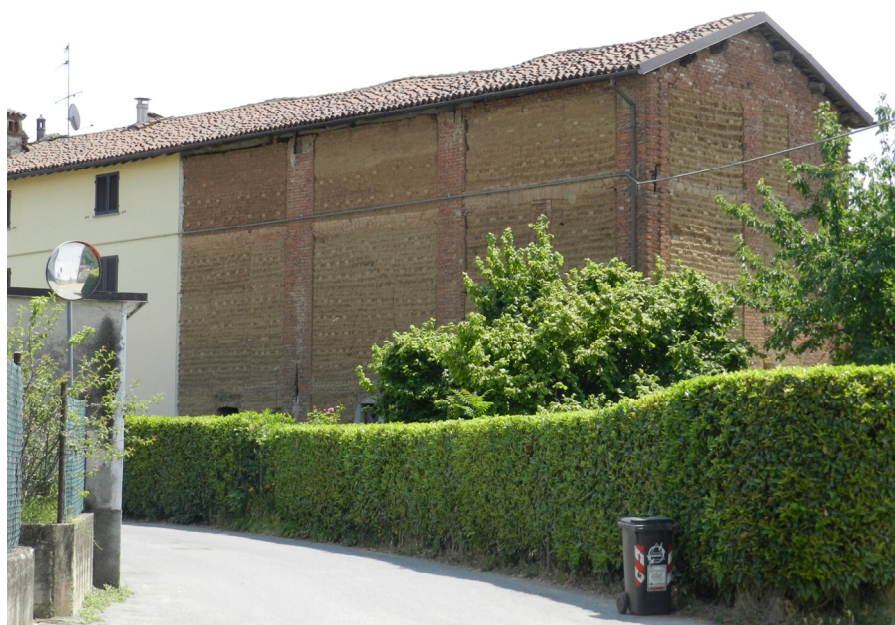
Figure 4. Vernacular earthen architecture in the Alessandria province, Piedmont, Italy (by Mattone, 2020).
