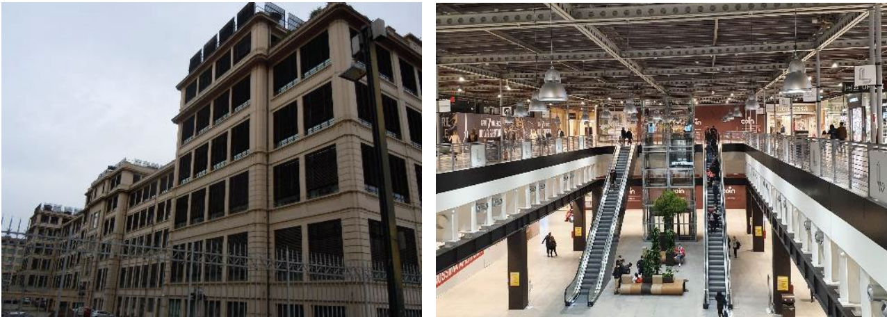
Fig. 6 - 7. Lingotto factory, Turin, Italy. 2003, end of the first multifunctional transformation (R. Maspoli) 2020, end of the extension of the shopping arcade (R. Maspoli)
