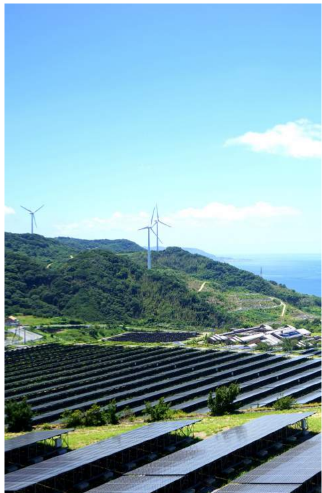
Solar and wind power station © Shutterstock
