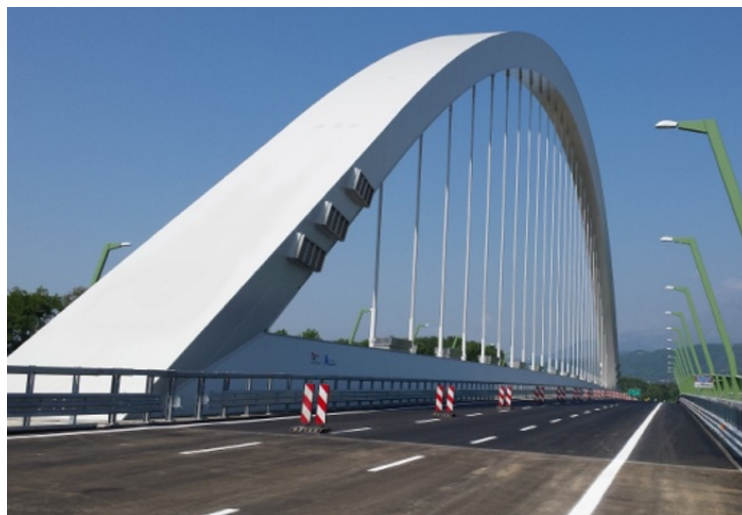
Fig. 2.1 General view of the viaduct
