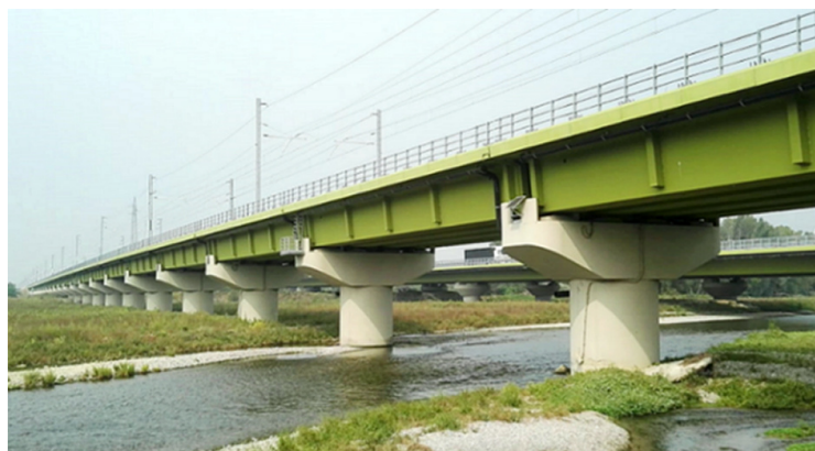
Fig. 3.2 General view of the Oglio Viaduct
