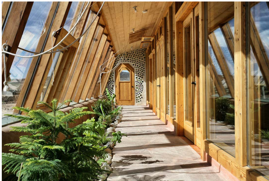
Figure 4. Passage used as a greenhouse within an earthship (Urbannext.net, 2022)
