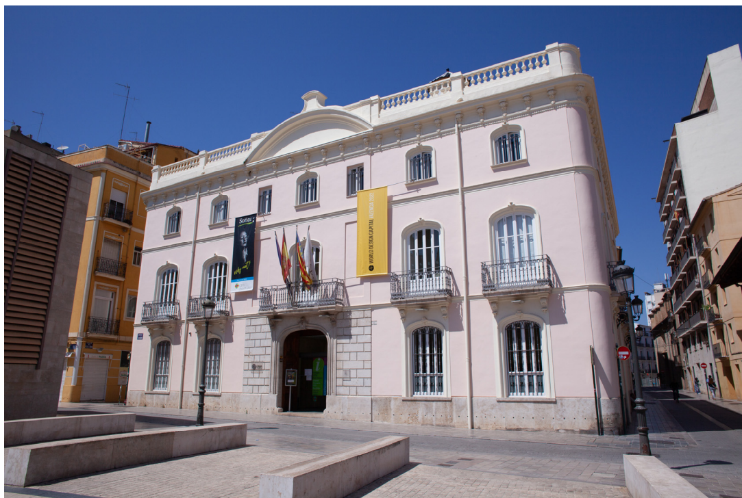
Figure 1. Colomina Palace (southern façade).
