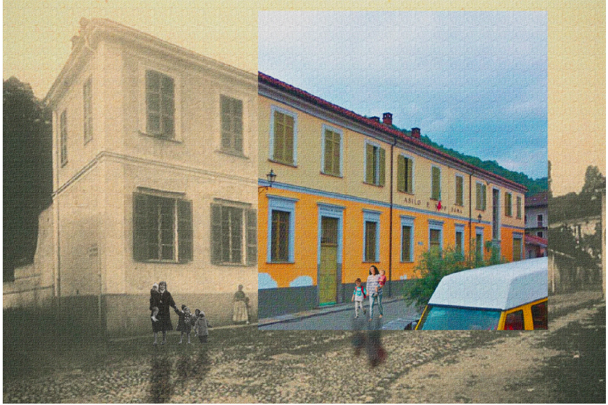
Fig. 7 | The kindergarten currently continues its activity and now serves the close municipalities.
