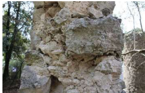
Fig. 11, 12. Details of castrum 's masonry (2021).
