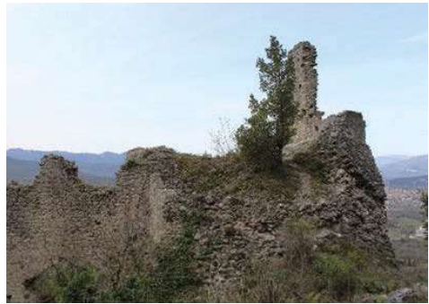
Fig. 7. External view of the keep (2021).
