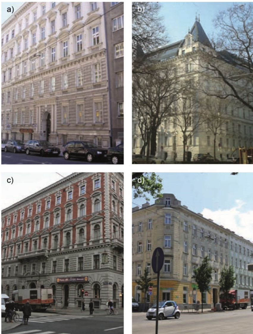
Figure 3. Overview of Gründerzeit buildings in the city of Vienna that undergone foundation soil treatment with expanding polyurethane resins.
