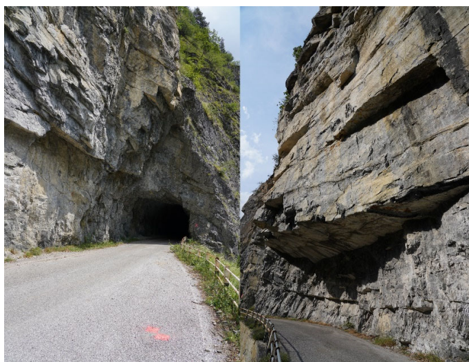
Figure 1. Photographs of the rock walls under study.
