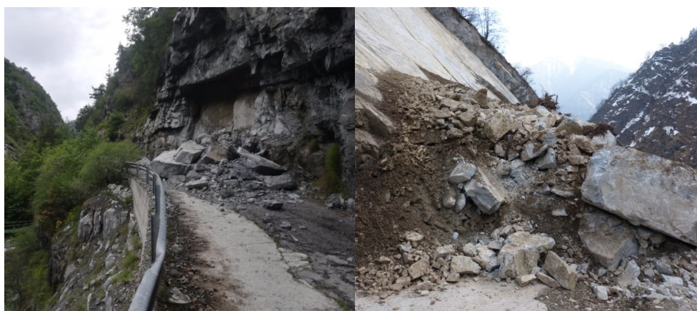
Figure 4. Instabilities of 2 June 2018 (about 250 \text{ m}^3 ) and 25 February 2015 (more than 2000 \text{ m}^3 ).
