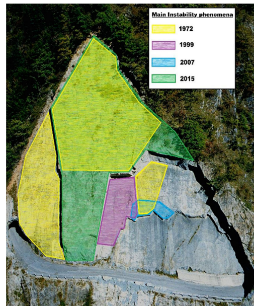
Figure 18. Chronology of the collapses in the LL sector (photo 2002).
