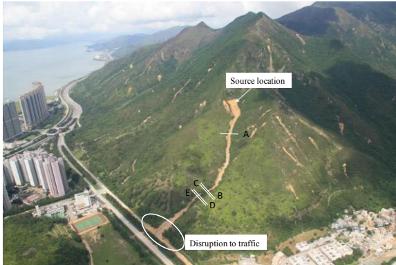
Figure 1. Yu Tung debris flow. The five sections indicate chainages (CH) where velocity estimates are available: A: CH100; B: CH413; C: CH439; D: CH462; E: CH477 (AECOM, 2012).
