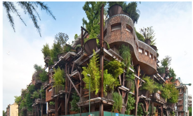
Fig. 4. The building "25 VERDE" in Turin, in Italy, designed by Luciano Pia architecture studio.
