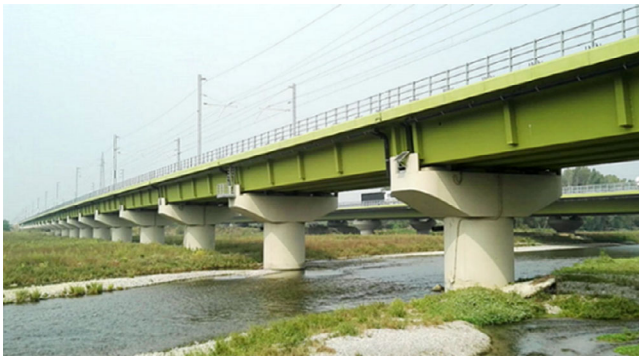
Figure 1. View of the Oglio Viaduct.
