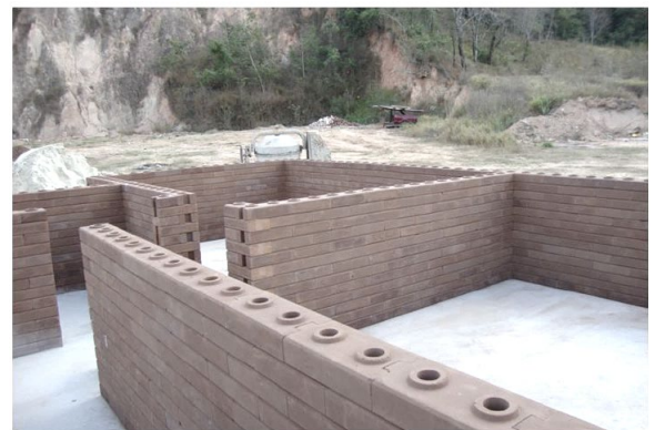
Fig. 2: Re-usage of tailings: civil structure made of iron tailings ([7]).
