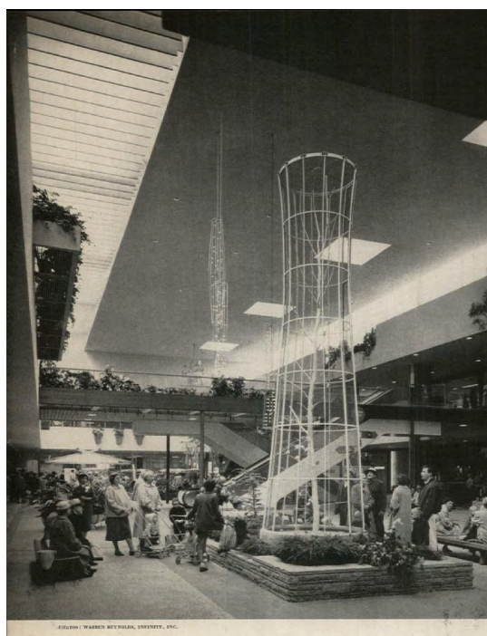
Fig. 4-5: Gruen & Krummeck. Southdale Shopping Center, Minneapolis, 1956.
