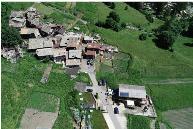
Figure 2. Aerial view of Pomieri hamlet case study.
