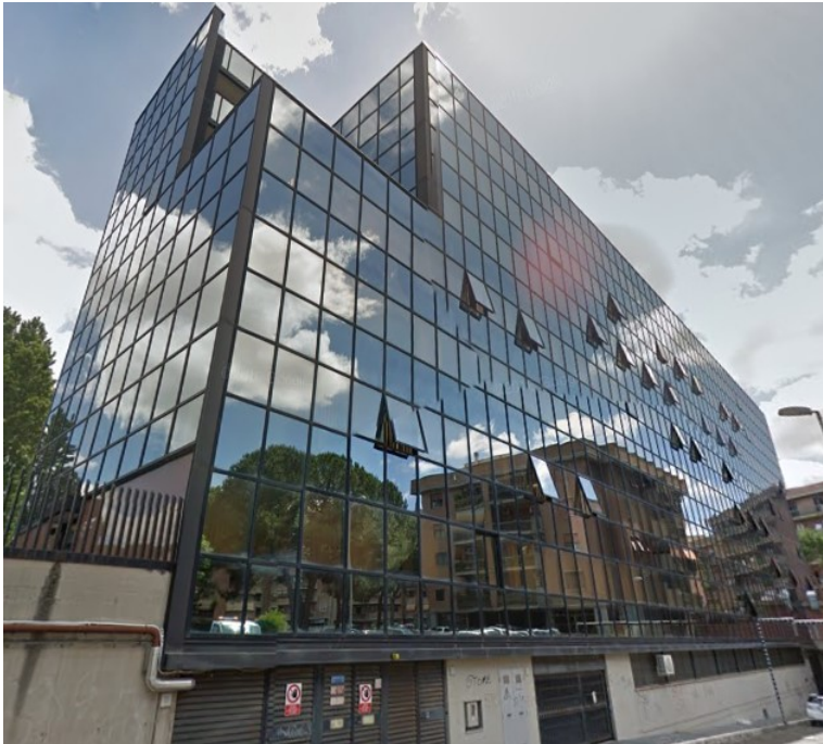
Fig. 2. Image of the building.
