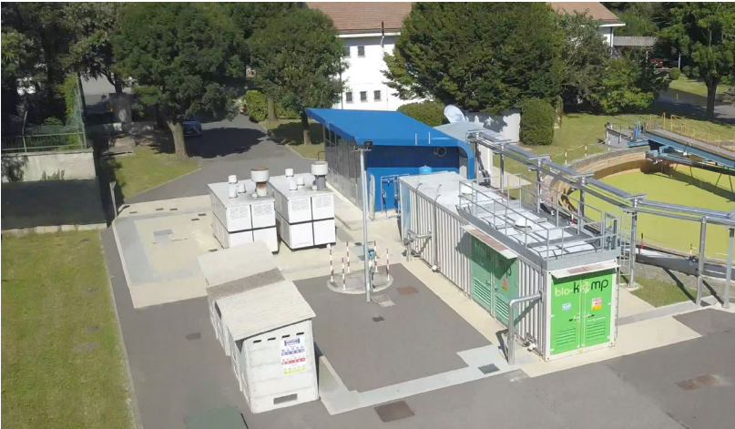
Figure 1. DEMOSOFC plant aerial view. The cleaning container is the grey and green 40 feet container one on the right.
