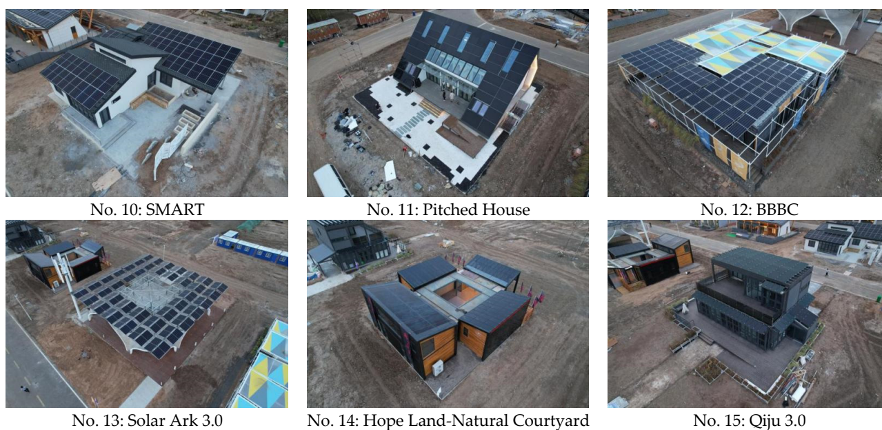
Figure 2. Buildings site photos.
