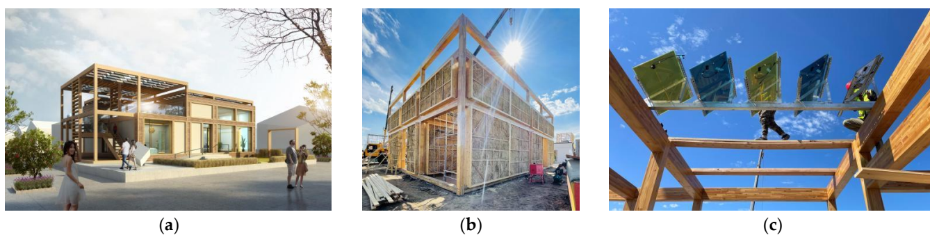
Figure 5. Main results of the Modular Sustainable Cube. (a) Straw bale modules. (b) Prefabricated materials. (c) PV panels.
