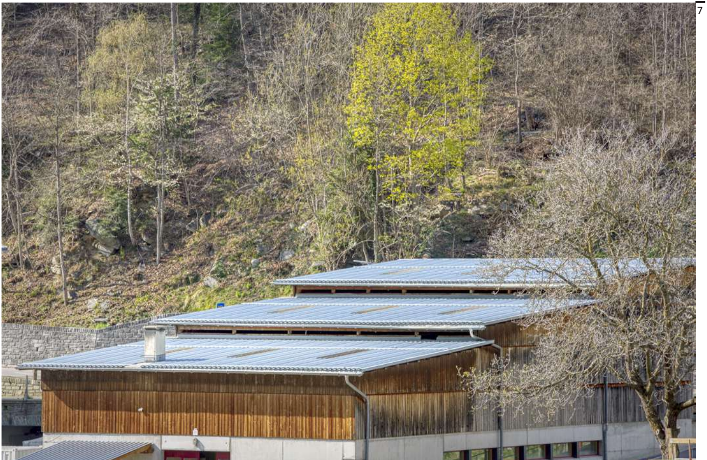
Fig. 7 The sequence of the sloping sheet metal roof.
