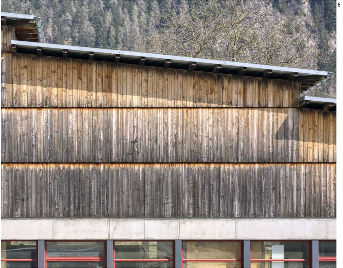
Fig. 7 The sequence of the sloping sheet metal roof.
