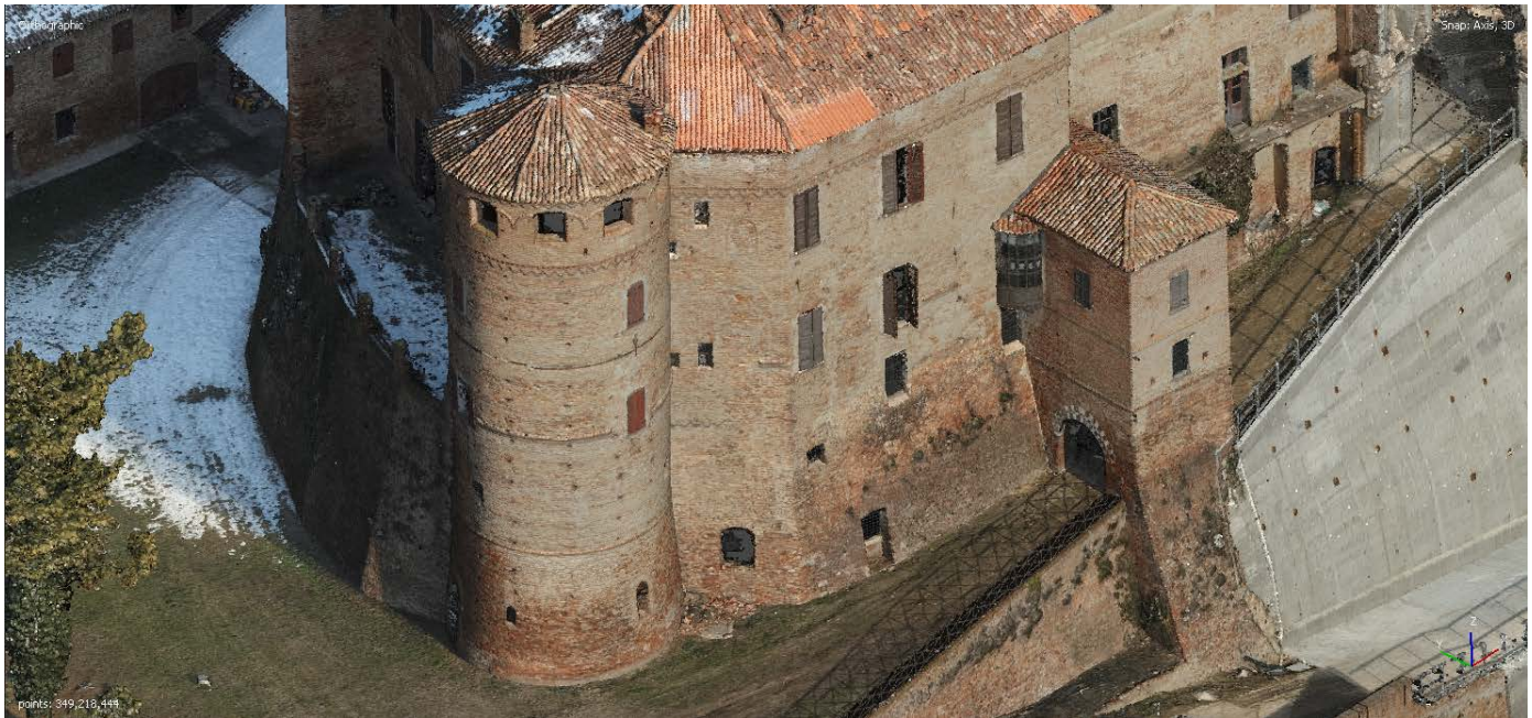
Figure 8. Photogrammetric output via Agisoft Metashape: detail on the east–west side of the castle and the circular tower (point dimension 1 pixel).
