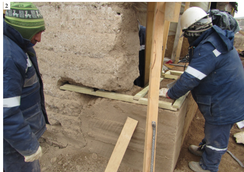
1: Process of reconstruction of a rammed-earth wall 2: Wooden reinforcement of a rammed-earth wall
