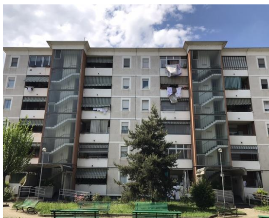
Figure 2. Photograph of the south-east elevation of the Reference Building.
