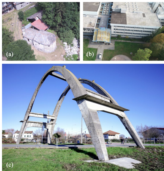
Figure 1. Case studies: (a) the rural chapel in Molini Allioni (Elva, Cuneo); (b) C. Alvaro-P. Gobetti Comprehensive School (Torino); (c) the parabolic arch of Morano sul Po.
