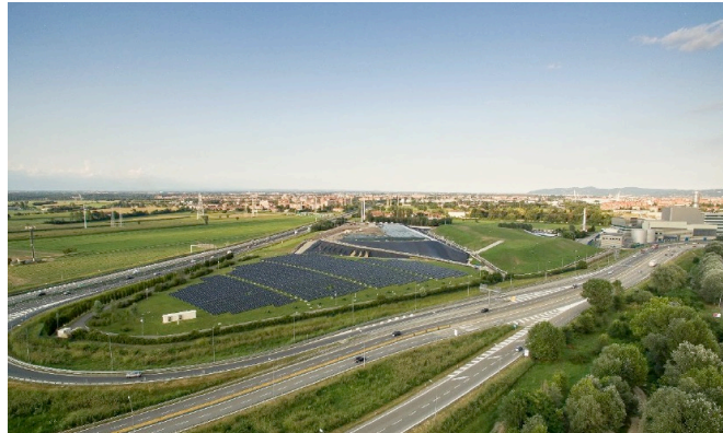
Figure 2. Photo of the Barricalla landfill.
