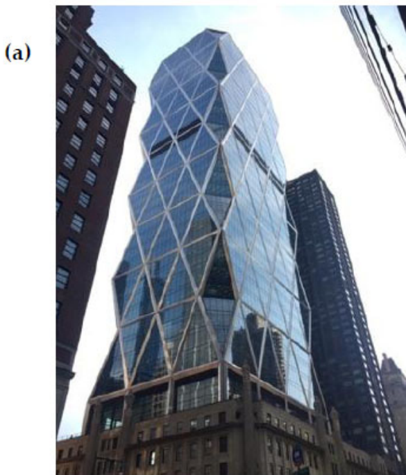
Fig. (2). (a) One of the first realized diagrid tall buildings: the Hearst Tower in New York City, NY, USA (picture taken by D. Scaramozzino); (b-c) number of research papers published about diagrids according to the SCOPUS database in the period 2005–2021 (data collected as of May 14, 2021).
