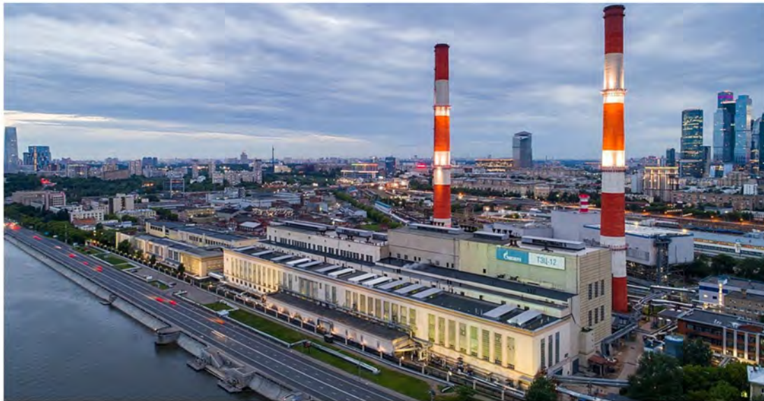
Figure 18. Moscow No. 12 Power Plant. (Source: [51]).
