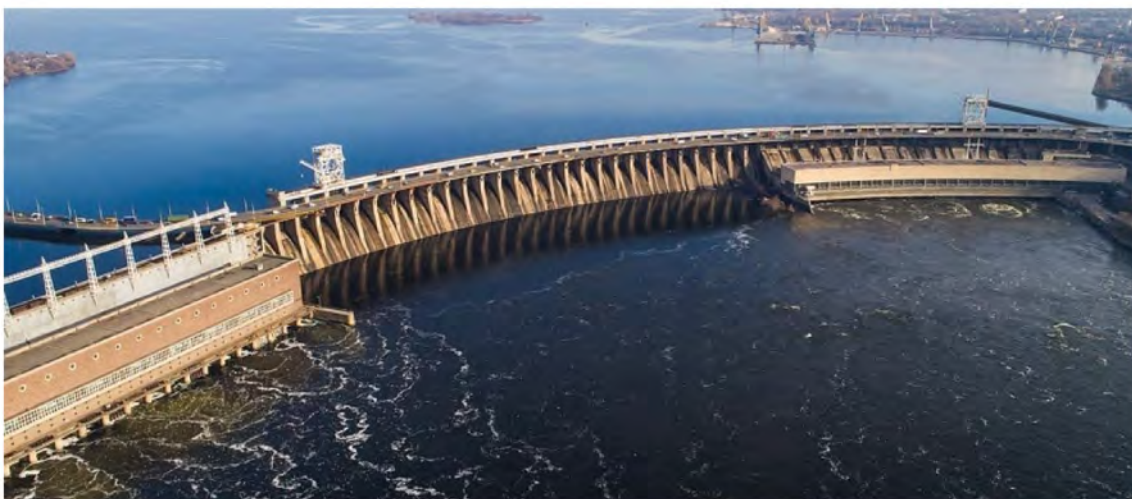
Figure 13. The dam of the Dnieper Hydroelectric Station. (Source: [40]).
