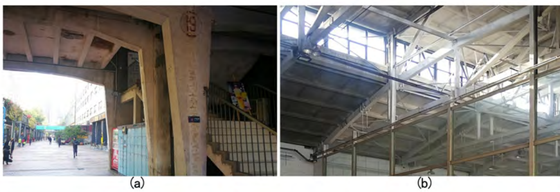
Figure 27. The Chengdu Hongguang Electronic Transistor Factory: (a) the reinforced concrete structure of Assembly Workshop (b) the steel frame roof truss of Testing Workshop.
