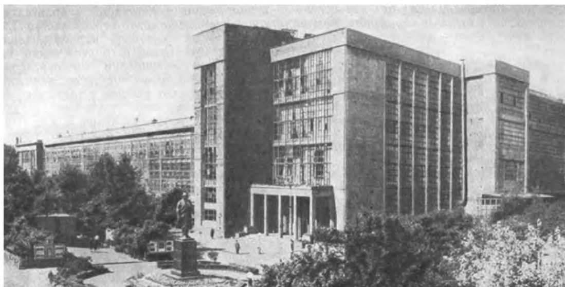
Figure 17. The new industrial building of the Moscow Stalin Automobile Plant. (Source: [45]).
