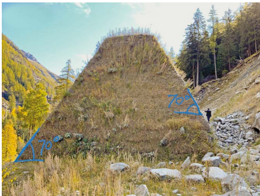
Fig. 1 – Reinforced earth rockfall protection embankments, Cogne, Valle d'Aosta Autonomous Region, Italy.
