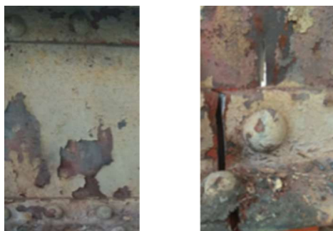
Fig. 2. Two different images from Quisi railway steel bridge
