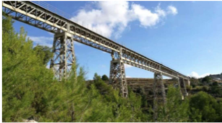
Fig. 1. Quisi (railway) steel truss bridge-Benissa
