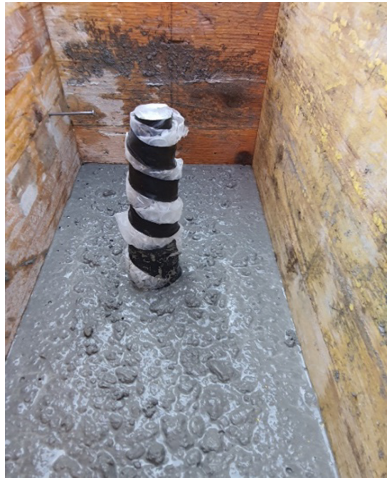
Fig. 3. Detail of the guided waves insulation during the casting in the framework of the concrete beam.
