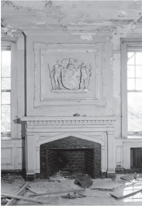
An original fireplace and mantle, the interiors of the building no longer exist, 1983 ( https://www.theruin.org/history ).
