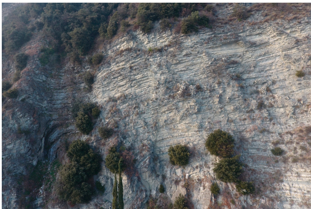
Figure 2. Rock face along the Gardesana Road (Italy).
