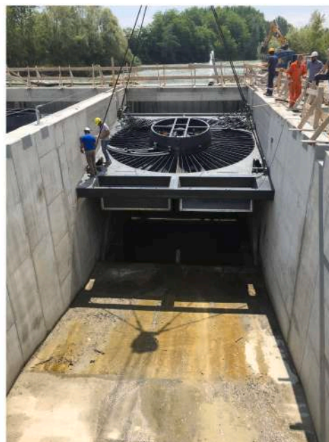
(b) Installation on the movable guide
