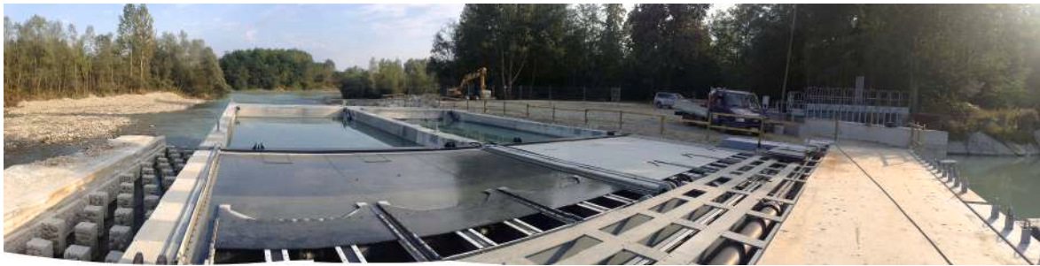
Fig. 15. VLHT installation in the canal, Mazzè, Italy.
