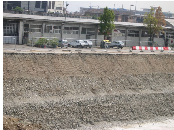
Fig. 17 - An approximately 15 m deep recent building excavation within Turin (Giordano Bruno Street, G in Fig. 14) shows the sequence formed by gravelly and sandy outwash sediments, supplied by the Dora Riparia River during the Upper Pleistocene.
