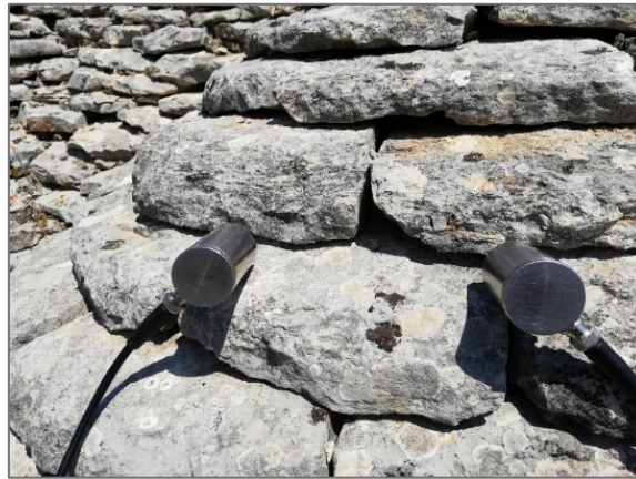
Figure 6: On site tests performed through UPV measurements on relevant cultural buildings, such as Trullo Palmullo, built in the first years of 1800 in Martina Franca. In this figure, a measurement is being taken on the cone of a trullo.
