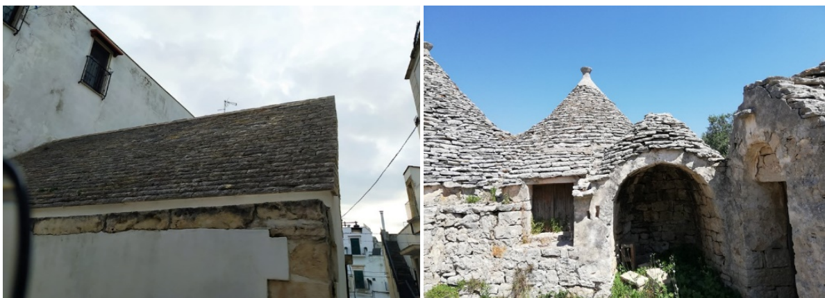
Figure 3: on the left) a modern building with sawn limestones replacing traditional chiancarelle of the roof (cortesy of arch. Intini 2020); on the right) a typical trullo in Itria Valley.
