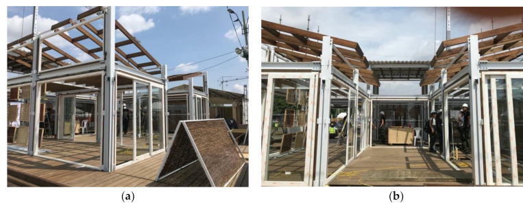
Figure 5. The PEI Maquina Verde’s House construction: (a) on the left the floor and the roof wood beam installation; on the right corner the shading device before the installation, it has made up with vegetal texture installed above a metal frame; (b) the PVC windows installation over the steel structure, the window-to-wall ratio is 80%.
