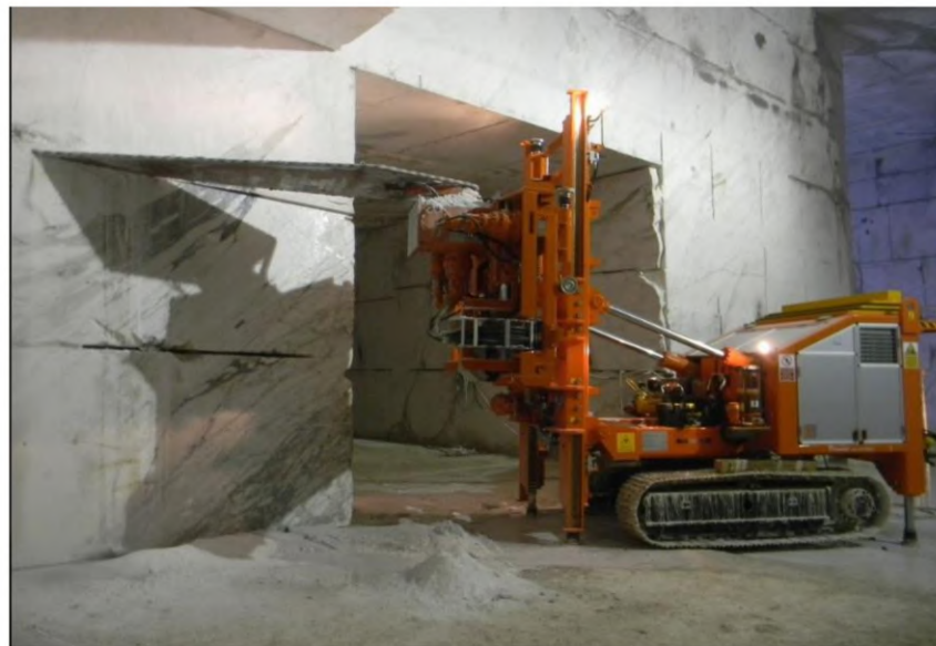
Figure 1. The chain cutting machine adopted in the quarry. The machine is engaged in a series of horizontal cuts to widen the underground opening (link https://www.fantinspa.it/en/gu70rxc-tunnel-chain-saw-machine/ , accessed on 2 October 2021).
