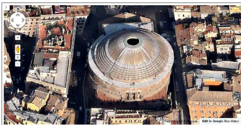
Figure 1 – The coffered concrete dome of the Pantheon in Rome, with a central opening (Oculus) to the sky, as seen from satellite (courtesy: Google Maps).
