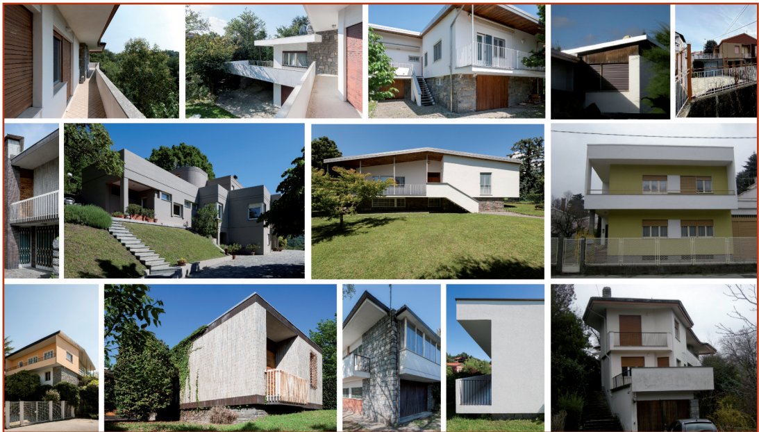
Figure 3 Some UCCD houses. Source: Paolo Mazzo's photos
