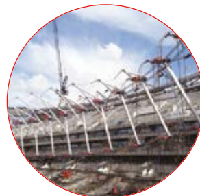
216 Strand Jacks working simultaneously
