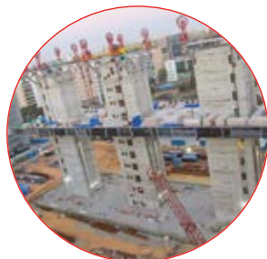
Installation of 10 complete Floor Slabs : Strand Jacks
