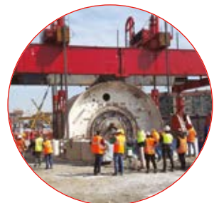
416 ton: Transport, Lowering and Installation
