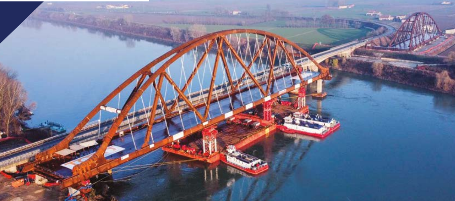
Transport and Installation of a 2,800 ton section of the new bridge San Benedetto Po in Mantova by means of barges, SPMTs, Tower lift and strand jacking system
