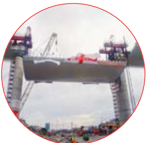
Installation of sections weighing up to 2,000 ton
