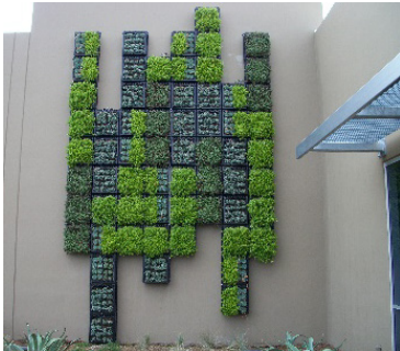
Fig. 3 Panel with soil substrate cells for planting
