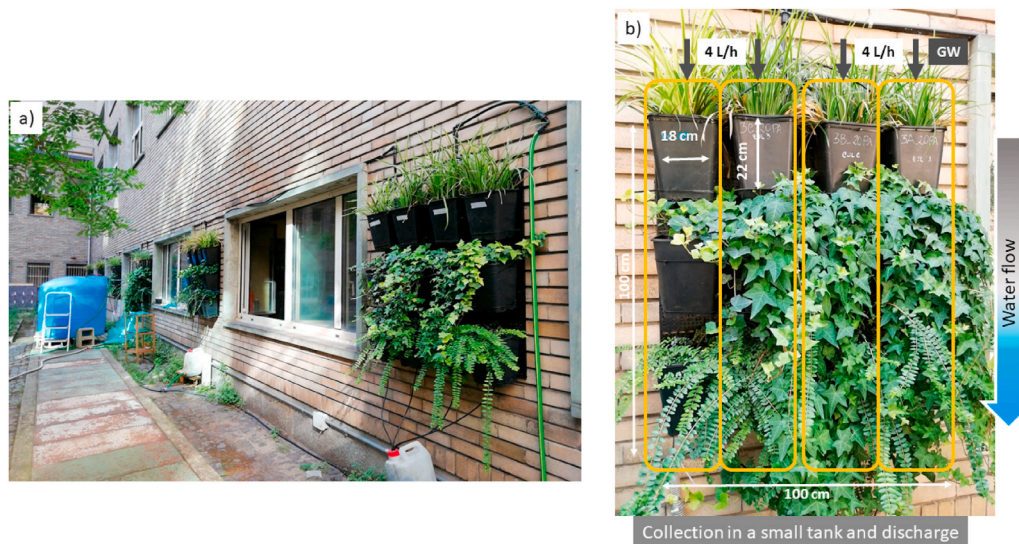
Fig. 1. a) Overview of the green wall panels; b) Detail of a modular panel. (For interpretation of the references to color in this figure legend, the reader is referred to the Web version of this article.)
