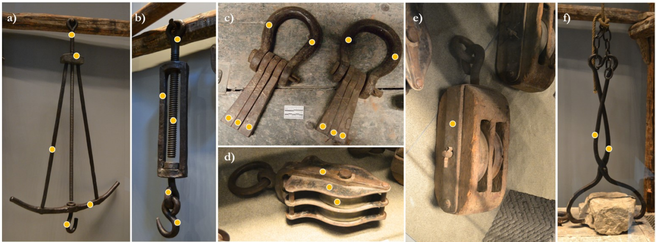
Figure 1. Historical tools employed for the construction of the Santa Maria del Fiore cathedral in Florence. The instruments are displayed in the Museo dell’Opera del Duomo, Florence: a), b) turnbuckles, c) three-legged lewises, d), e) pulleys, f) pincers. Yellow circles indicate the analyzed areas.
