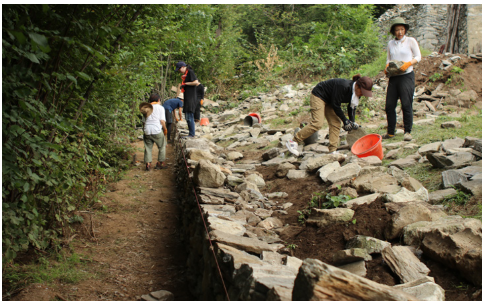
Construction activities during the 2019 workshop (Maurizio Cesprini)
