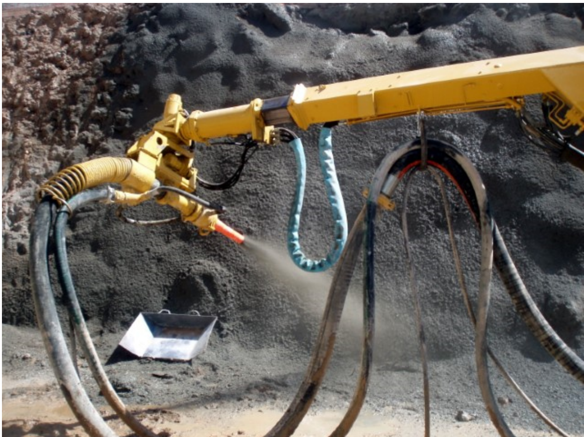
77 Fig. 1 Application of shotcrete
