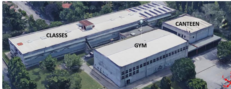
Fig. 1 – Structure overall view
