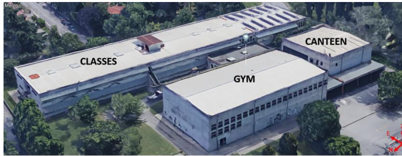
Fig. 1 – Structure overall view
