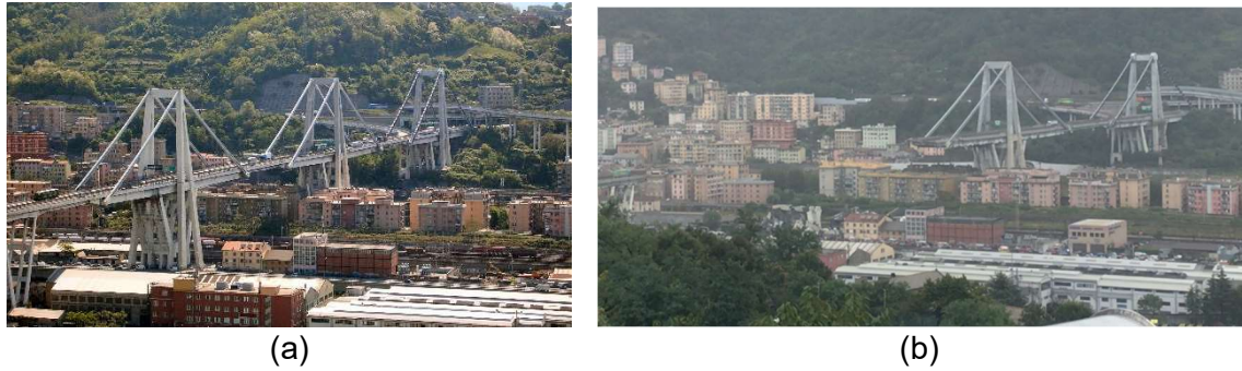
Figure 3: (a) Polcevera Viaduct in Genoa by Riccardo Morandi (Licensed under the Creative Commons Attribution-Share Alike 3.0 Unported license. Author: Bruno). (b) The collapse of Pier #9 (Licensed under the Creative Commons Attribution-Share Alike 4.0 International license. Author: Salvatore1991). The replacement bridge is open to traffic.
