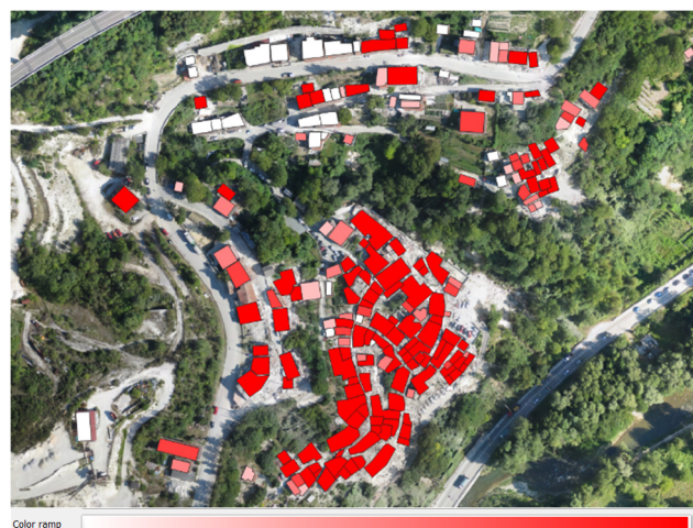
Figure 7. Damage classification performed by DEEP on the Pescara del Tronto 2016 orthophoto, using the new classification model based on the central Italy earthquake dataset. The color scale shows the classification likelihood score of belonging to the "not damaged" class (0 - in white) or to the "damaged" class (1 - in red).
